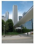
To determine whether it could support the Nichols Bridgeway, WJE evaluated the strength of the Millennium Garage roof, designed bridge piers and roof strengthening solutions, and prepared construction documents for the bridge's foundation system. WJE provided on-site observation and troubleshooting during construction to ensure a successful outcome.
