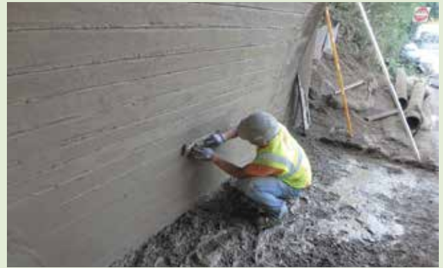
Finishing form-board lines in wet shotcrete
