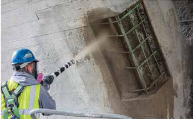
Fig. 8: Dry-method shotcrete repair on arch rib corner
