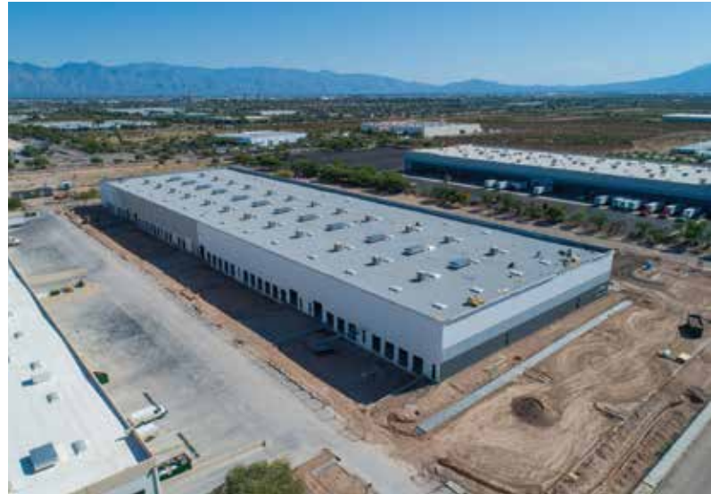
Figure 1. Concrete or masonry wall “big box” building, a common occurrence of the building type addressed by the alternative RWFD design method. Credit: Schnitzer Properties/VLMK Engineering + Design.
